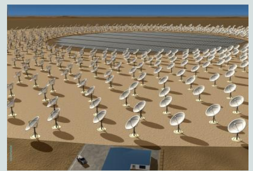
A visualization of the SKA core site. Small dishes will receive short radio waves while static. Credit: CSIRO Australia
